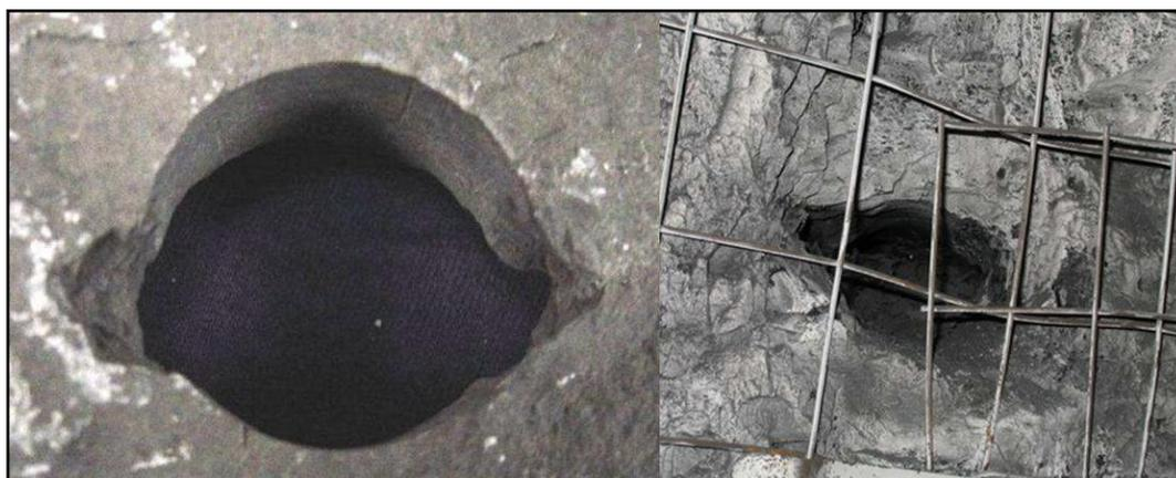
Figure 1: Examples of borehole breakout.
