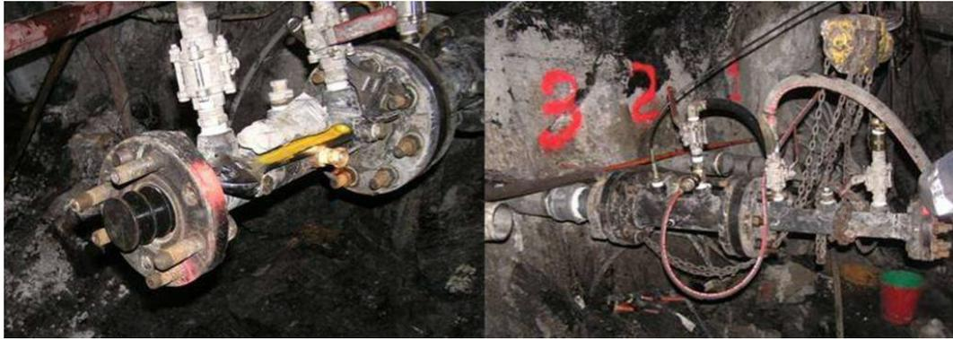
Figure 2: Displacement plug and cement head used during cementing.
