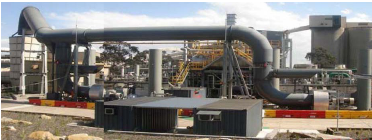
Figure 9: West Cliff Colliery mine ventilation air methane abatement and utilisation plant – WestVAMP
